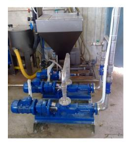
**DN pump**DN series used for transfer of polymer and sludge in a waste water treatment plant.
