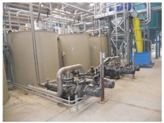
**DN pump**DN series used for chemical thickened sludge transfer to centrifugal treatment.
